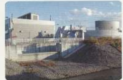
No. 4 bank (Overflow levee)
