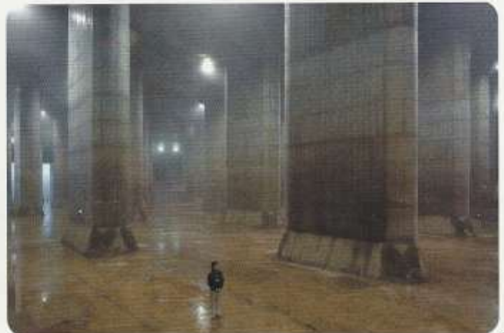
Pressure-adjusting water tank
