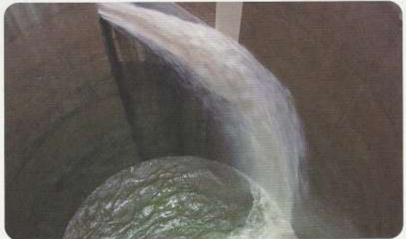
No. 5 bank (State of inflow)
